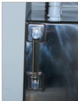
Figure 7. Tube on large holding tank for visual inspection.
